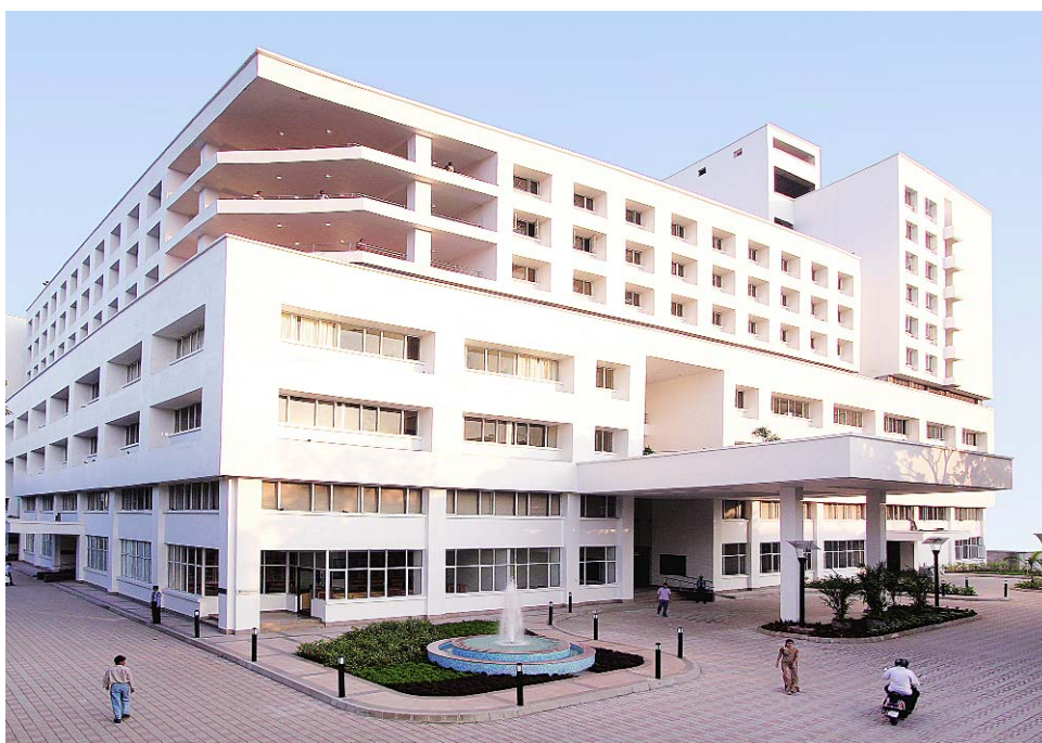
Jupiter Hospital's Thane facility with 350+ beds across seven floors
